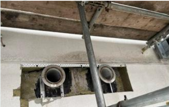
A photo showing Phase 1 South Elevation – Stainless steel sleeves installation works to EWI areas progressing
