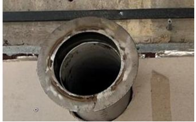
A photo showing Phase 1 South Elevation – Stainless steel sleeves installation works to EWI areas progressing
